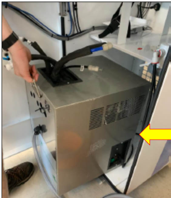
SU V0.75: Ice Bank Fill Valve - (Chiller lines coming from the Top)
