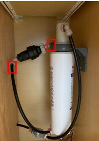
NOTE: Waterblock is horizontal for illustration purposes, should be installed vertically
