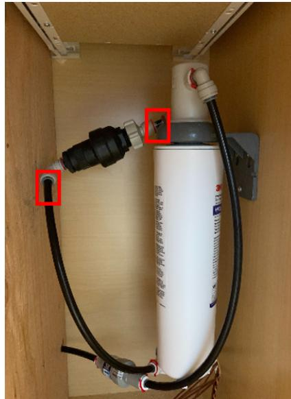
**NOTE: Waterblock is horizontal for illustration purposes, should be installed vertically**
