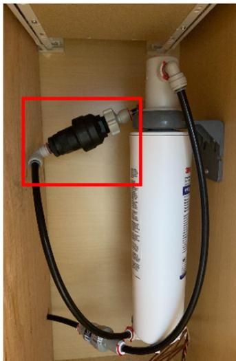
**NOTE: Waterblock is horizontal for illustration purposes, should be installed vertically**
