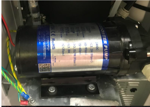
Demand Pump - Found by removing the mid back panel, on the plumbing shelf
