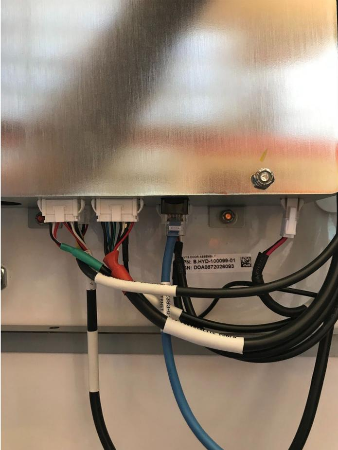
4. Remove the (4) screws (2 on top and 2 on bottom) securing the display and control box to the door using a  $\frac{3}{8}$ " socket wrench.
