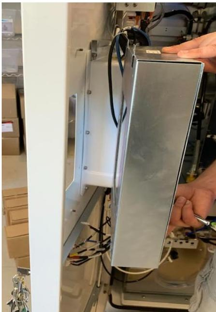
6. Replace the old display and control box with new assembly.
