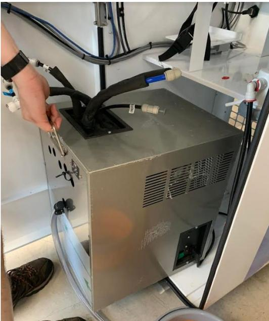
9. Remove the power plug from the side of the carbonator.
