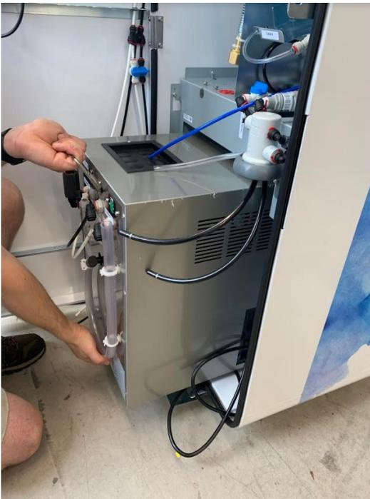
14. To re-install the carbonator, perform steps 1-13 in reverse order, omitting the water line purges and emptying the carbonator.
