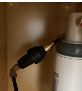
NOTE: After reinserting the waterblock, the tube markings created earlier should be visible at the edge of the fitting
